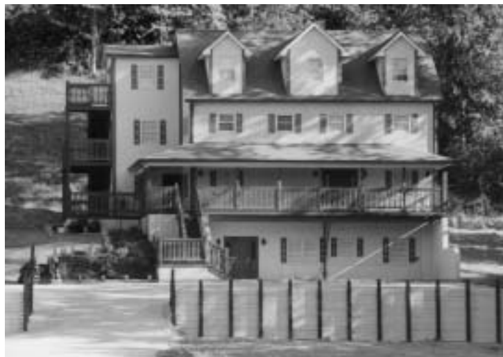
The new shelter was made possible with a $500,000 federal grant. The two-year-old building will have 10 bedrooms, a playroom as well as offices for staff.
